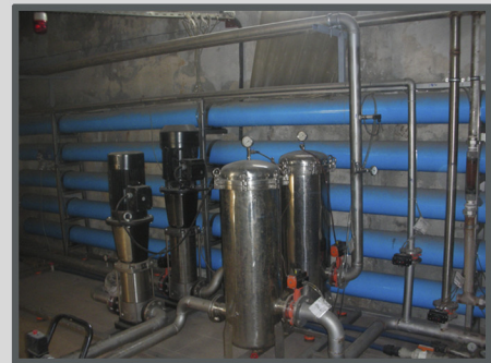
Reverse Osmosis Facility for Reducing Water Usage
